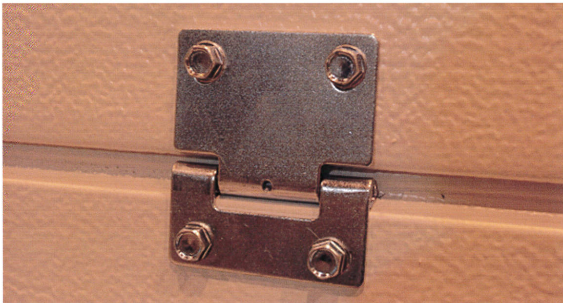
Figure 4. Intermediate hinge.
